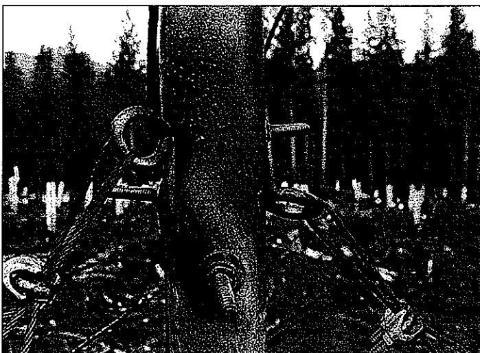
Figure 3. Guy wire attachment.
